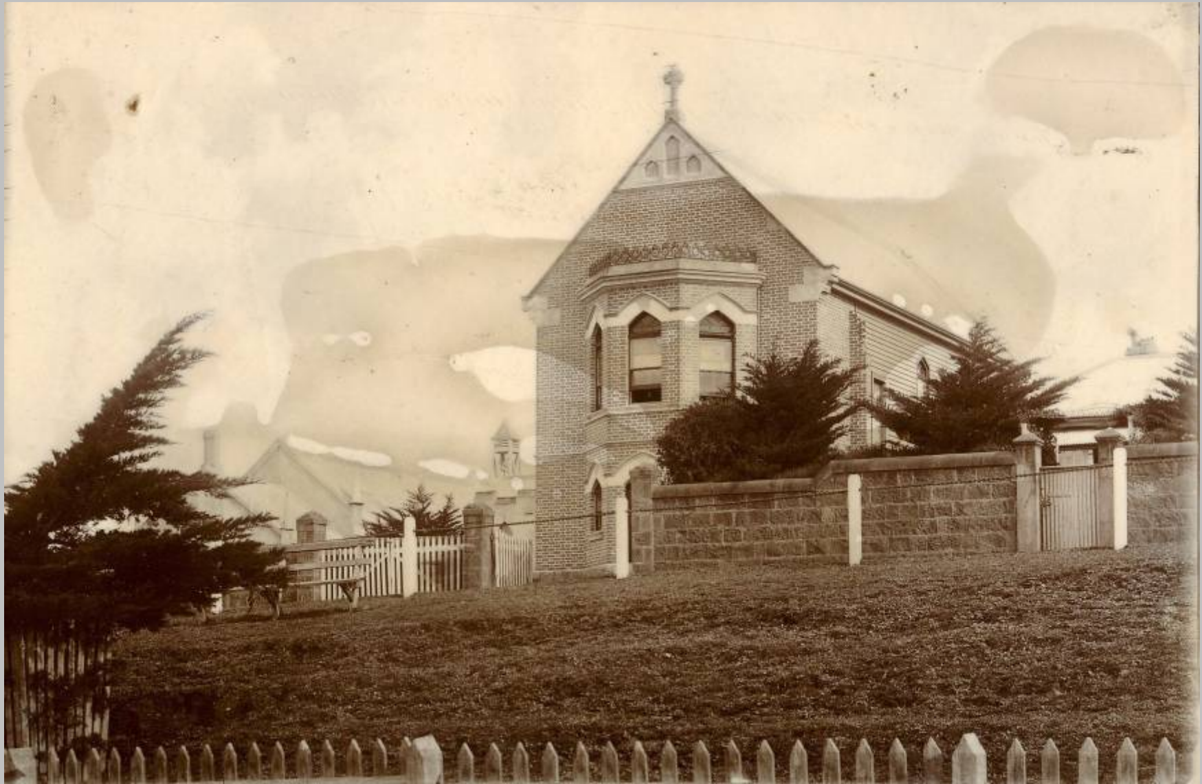
Portland Convent, 1900, with the new wing built next to Bayview Cottage comprising dormitory and school room. All Saints School on the left and All Saints Church on the far left.
