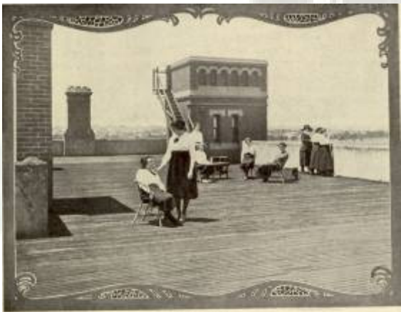
On the flat roof of the Albert Park Convent, opened in 1890 and including the Central Catholic Teachers' Training College in 1906
